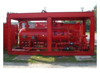
Three phase, horizontal, H₂S service separators "E-I" and "E-II"
